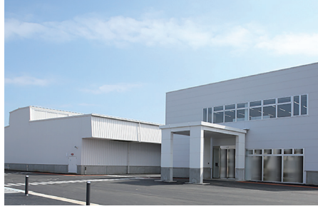
Opened Shiroi Data Center Campus (2019)
