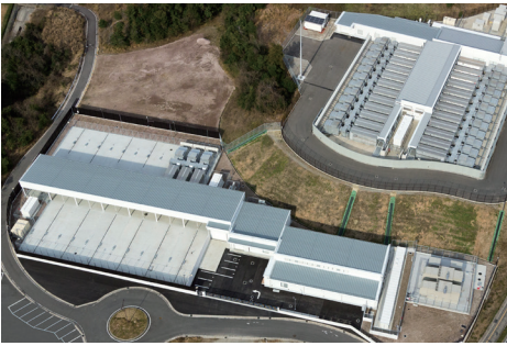
Opened Matsue Data Center Park (2011)
